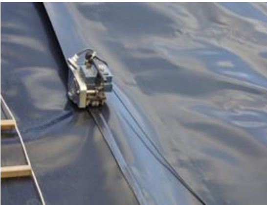
HDPE Sheet Welding
