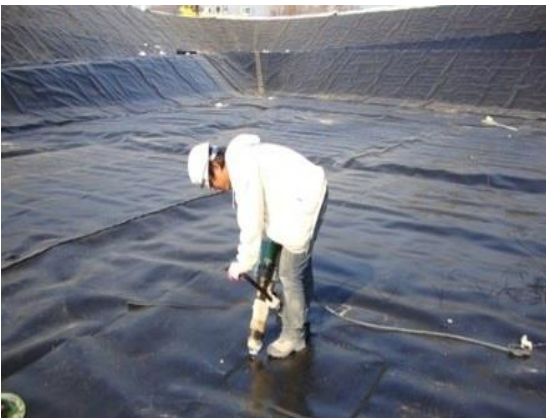
Repair & Vacuum Test
