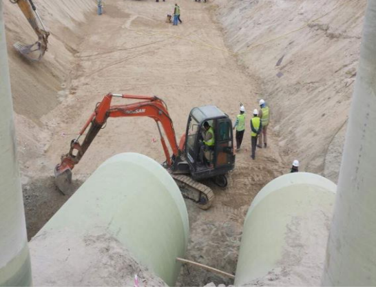
GRP Pipe Laying
