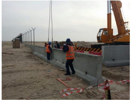
Fence Work in Progress
