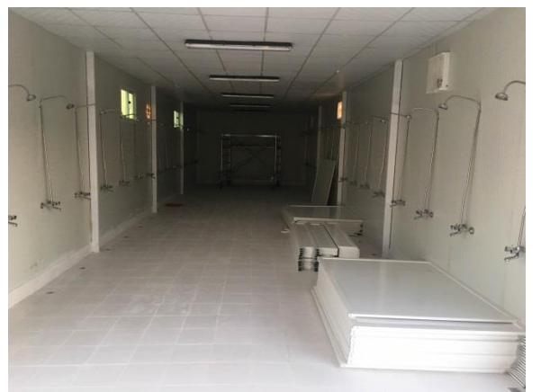
Interior Works in Toilet Block
