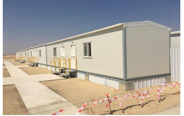
Exterior of Toilet Block
