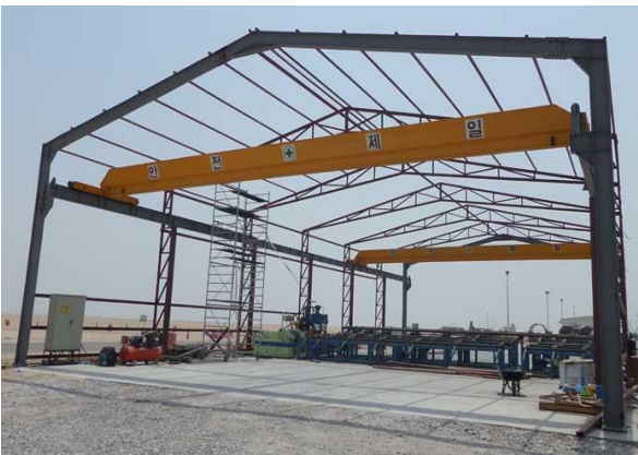
Heavy Structural Erection Work
