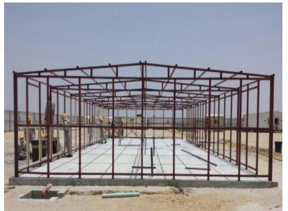
Light Structural Erection Work
