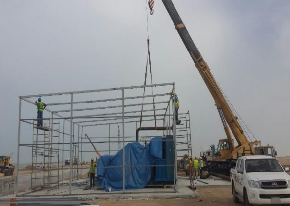
Structural Fabrication work
