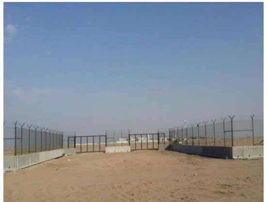
Finished Fence Work
