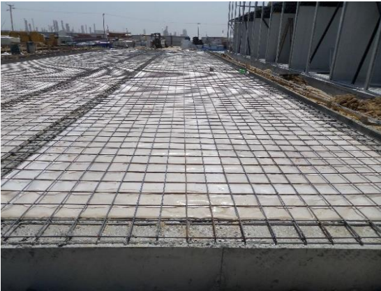
RCC Floor Construction
