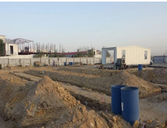
Preliminary site Preparation Work
